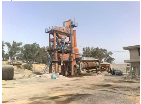
Fig. 2 An example view of small-scale asphalt plant in Iran
